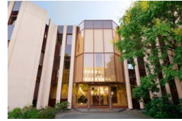
Pully (VD) 1 Avenue Charles-Ferdinand Ramuz 43
